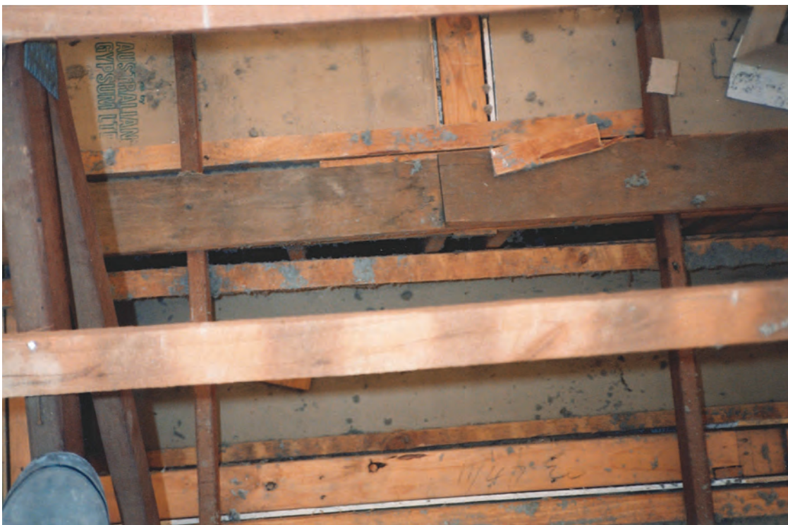
Figure 5 – roof space during remediation (note gap to wall cavity)
