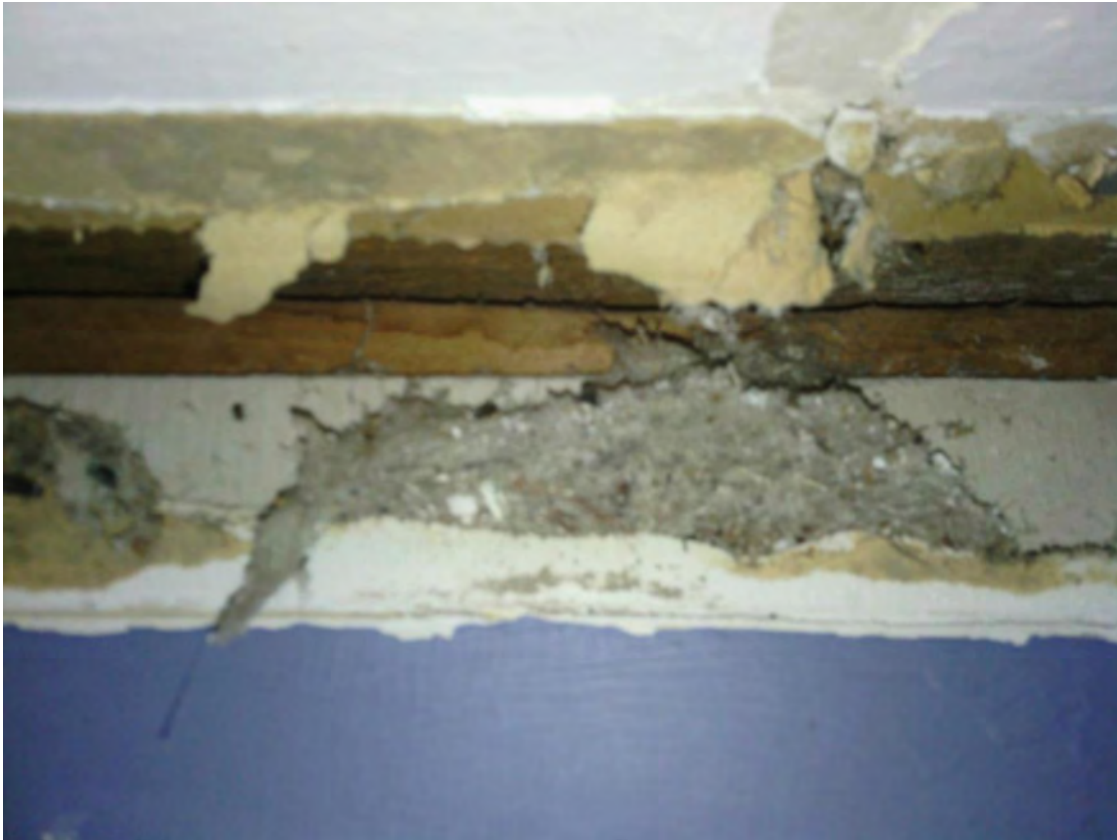
Figure 7 – asbestos in an internal wall
