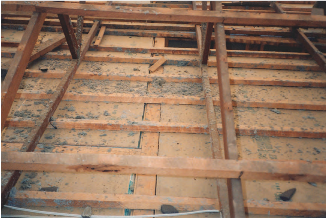
Figure 5 – roof space during remediation (note gap to wall cavity)
