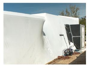
The other method involves using shrink wrap to encapsulate the entire house.
