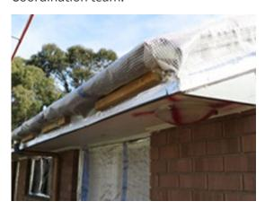
One method involves placing plastic sheeting on the roof and sealing all windows and vents.
