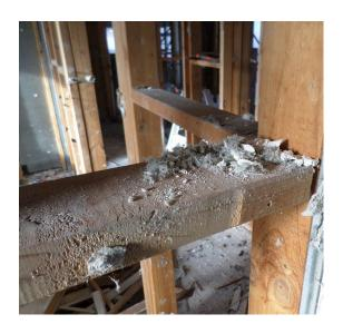
Under negative air conditions the house is deconstructed internally. Ceilings and walls are pulled away to expose the cavities where loose fill asbestos insulation fibres have settled.
