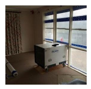
Once the houses are sealed, negative air pressure units are placed in windows or doors.
