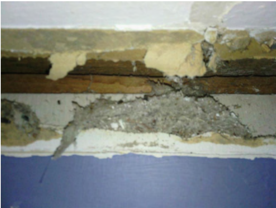
Figure 7 – asbestos in an internal wall
