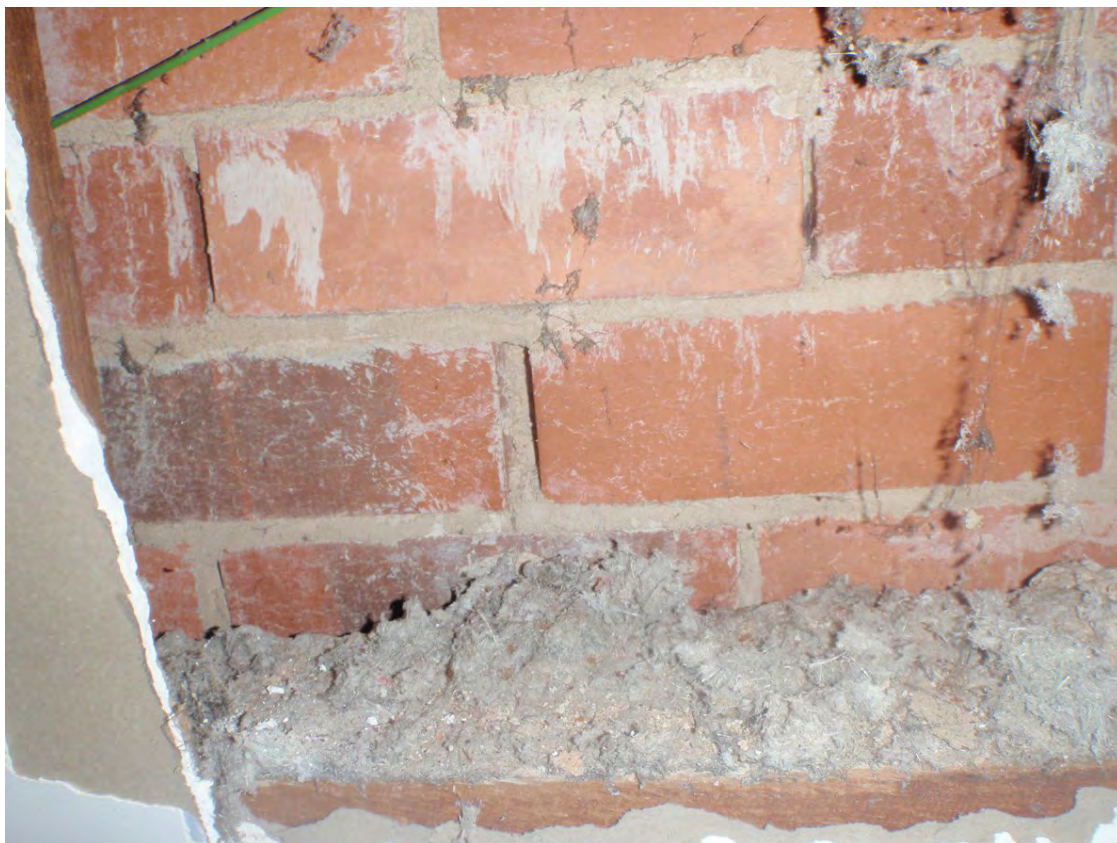
Figure 1 – asbestos in an external wall (of an unremediated home)
