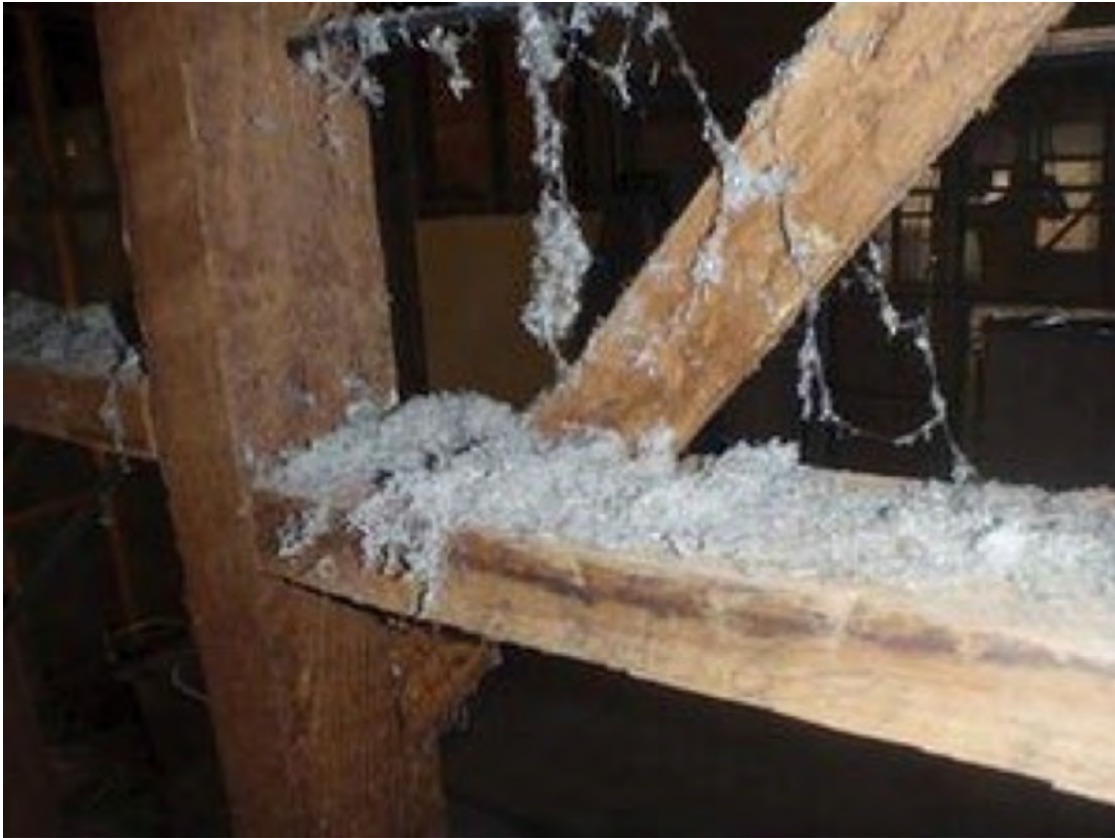
Figure 2 – asbestos in an interior wall (note new cable penetrating stud at top left)
