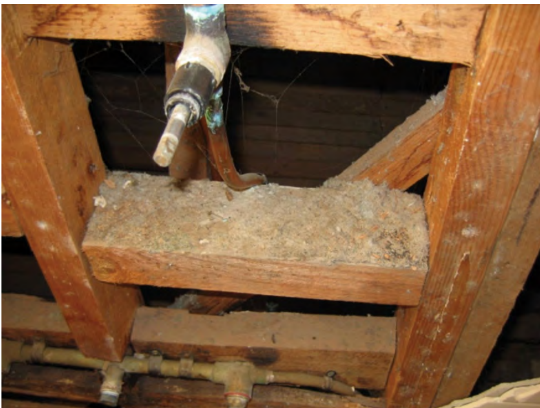
Figure 7 – asbestos in an internal wall
